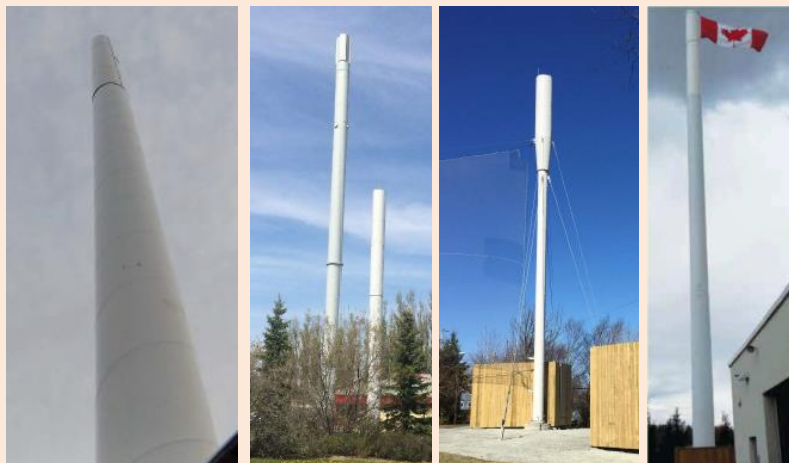
The above images show examples of smooth, shrouded monopoles and flagpoles that should be considered at risk of Vortex Shedding vibrations.
